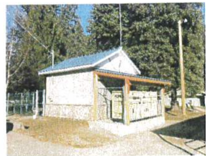
Sayward Well House & Generator
