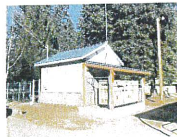
Sayward Well House & Generator
