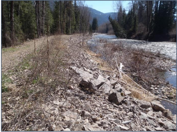
Photo 5. Mixture of cobble and boulder size angular rocks on face of dike.
