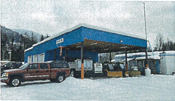
Building from NW
