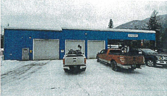
Building north side
