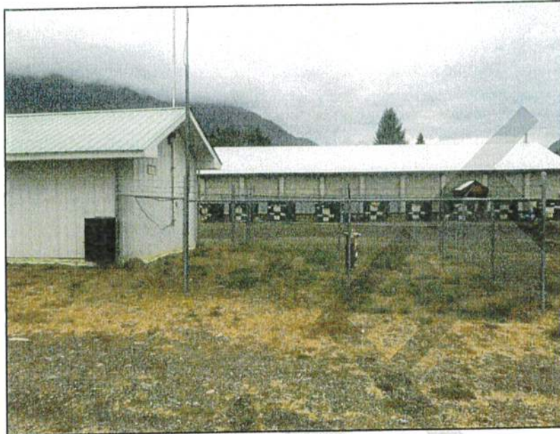
Photo 7: Glendale Well and Pumphouse (facing east)
