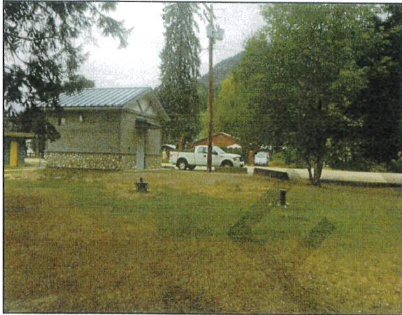
Photo 1: Sayward Well and Pumphouse (facing northwest)
