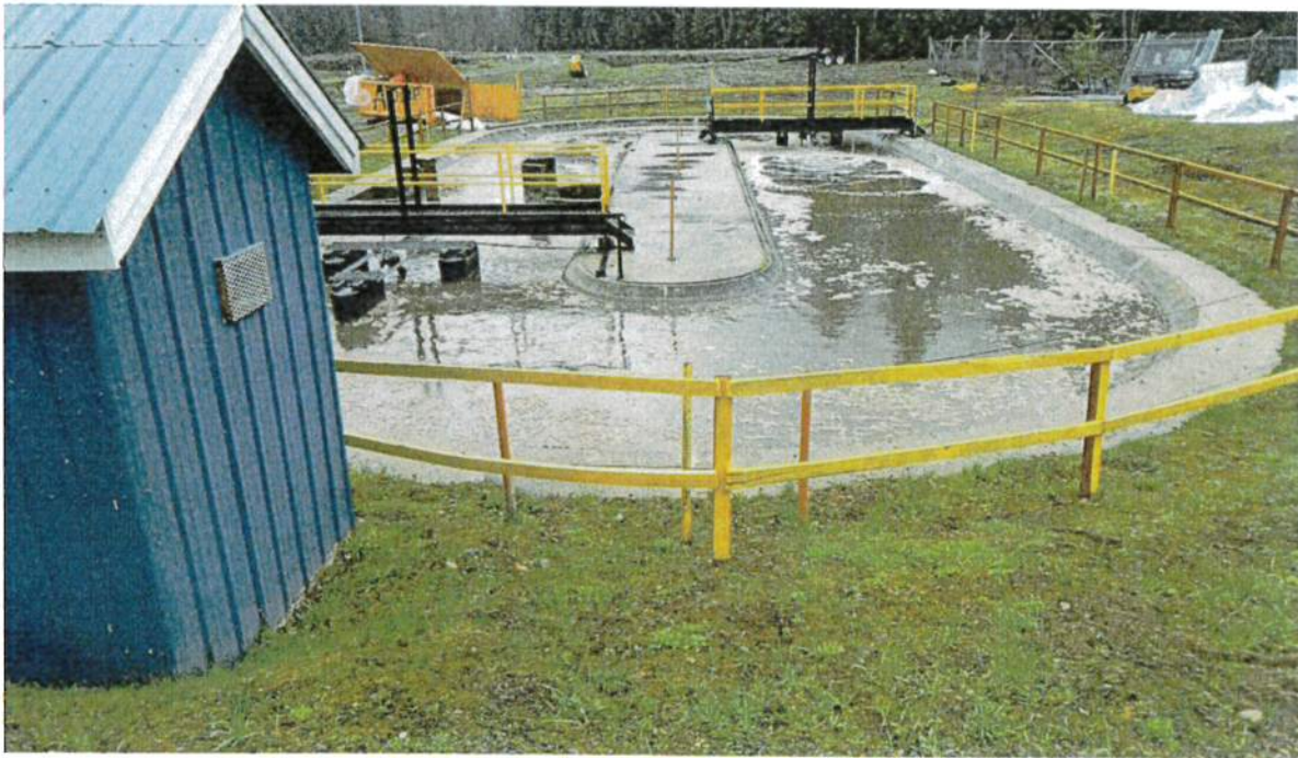
Wastewater Treatment Plant
