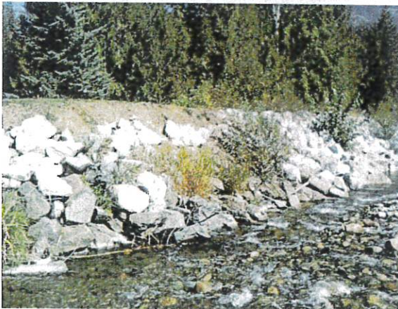
Location 5 – Slumping Lock Blocks and Shifting Armour
