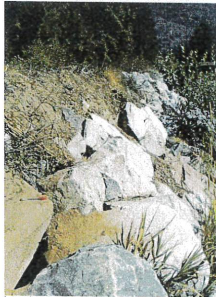
Location 5 – Slumping Lock Blocks and Shifting Armour
