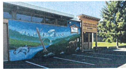
Salmo Valley Youth & Community Centre Building
