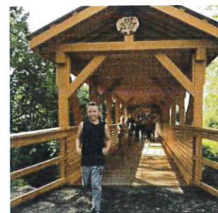
6 th Street Pedestrian Bridge
