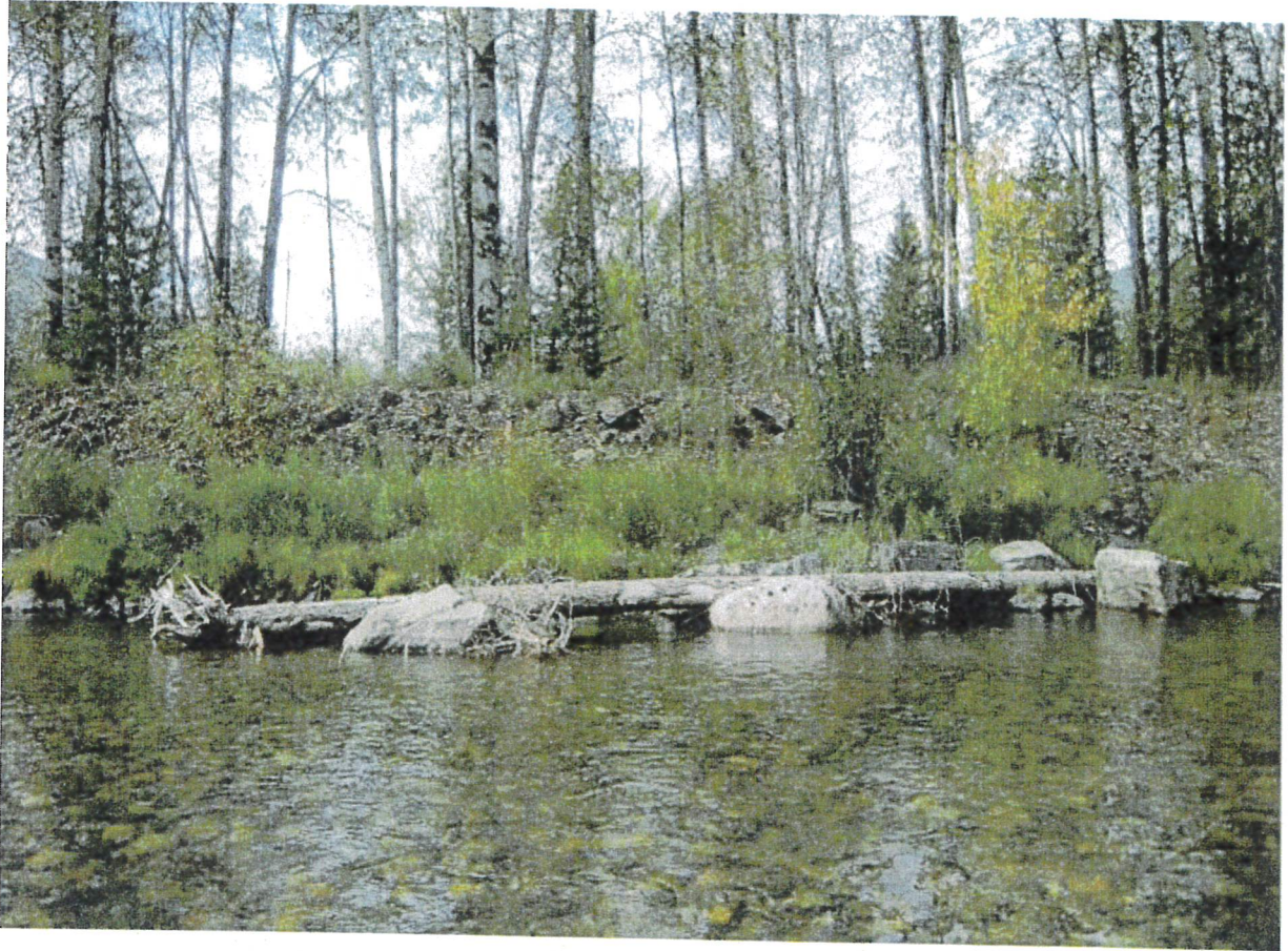
Cover photo: Lateral log LWD structure installed on bank of Salmo River upstream from study area.
